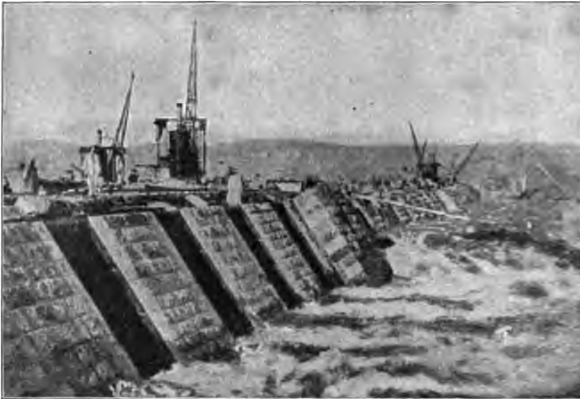
GREAT DAM ACROSS THE NILE—UPPER EGYPT.
